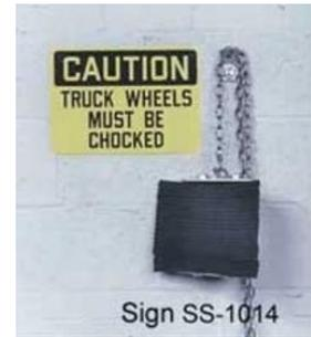
Prevent accidents at the loading dock. Lights and signs are used to aid truck drivers with dock safety procedures.
